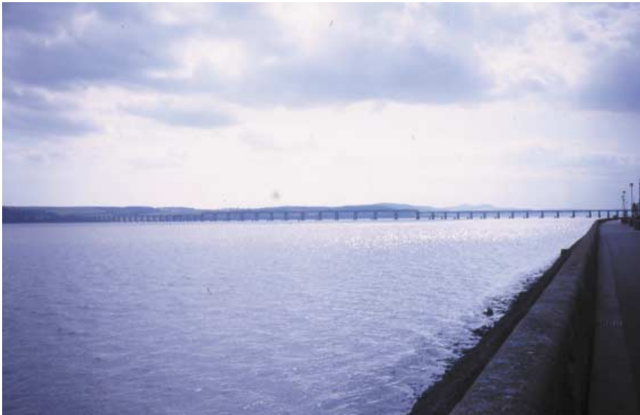
Fig. 3 The new Tay Rail Bridge, looking upriver (west) from Dundee, 27 July 2004 (note the stumps of the old bridge pillars at the water's surface and the new 'high girders') (© P. J. A. Burt)
